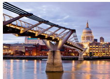
(c) Millenium Bridge, London (2000)
