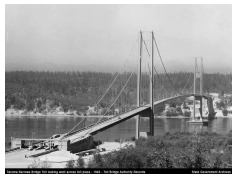
(b) Takoma Narrows Bridge, Washington (1940)
