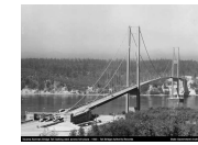
(b) Takoma Narrows Bridge, Washington (1940)
