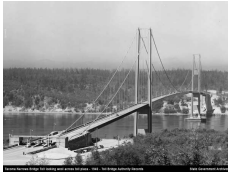
(b) Takoma Narrows Bridge, Washington (1940)
