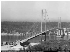
(b) Takoma Narrows Bridge, Washington (1940)
