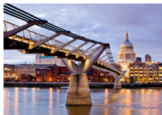
(c) Millenium Bridge, London (2000)
