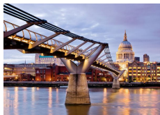
(c) Millenium Bridge, London (2000)
