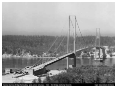
(b) Takoma Narrows Bridge, Washington (1940)
